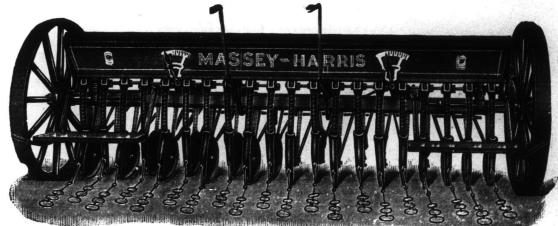
Made with 16, 20, 22 and 24 Shoes, Single and Double Discs. Frame Carries any Style Bottom.
