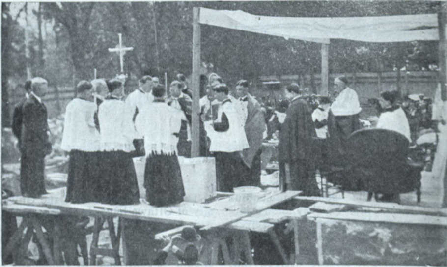
LAYING THE CORNER-STONE OF THE NEW ARTS BUILDING OF OTTAWA UNIVERSITY ON MAY 24TH
