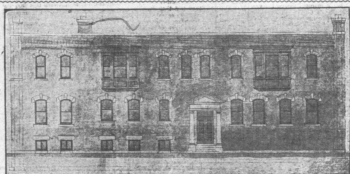
DALLAS ROAD FRONTAGE OF THE DETENTION SHEDS.
