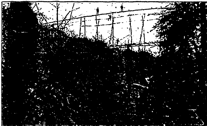
TRESTLE SUPPORTING LUMBER SLUICE OVER HUMMING BROOK, N. S.
