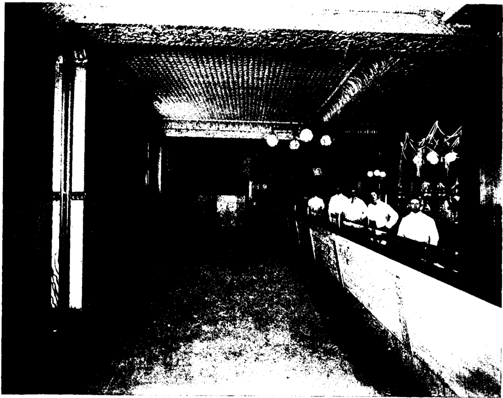
Interior of the newly remodeled Hotel Aberdeen, corner of Chestnut and Queen streets. Mr. McMillian, proprietor. Note the side wall, coping and floor, including base, is of the Hygienic Roman composition.
