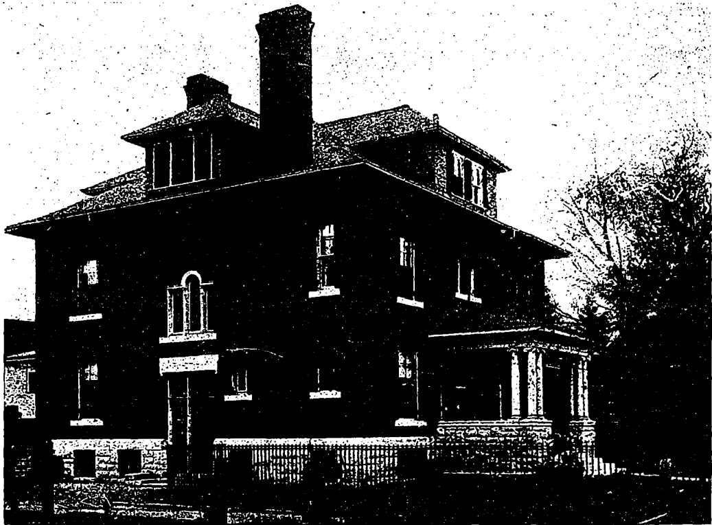
Residence of Architect John Woodman, River avenue, Winnipeg. A recent example of the square type of house which has a number of noteworthy features to commend it.
