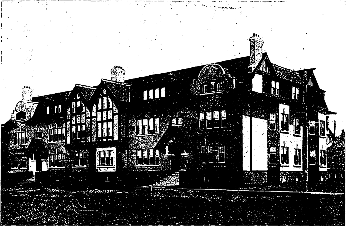
Albert Court Apartments, Regina. In exterior construction and architectural treatment this structure stands out in marked distinction to the usual type of apartment buildings. There is a strong domestic feeling in general lines, and a pleasing color contrast in the buff tones of the stucco walls, brown woodwork and red shingle roof. Storey & Van Egmond, Architects.
