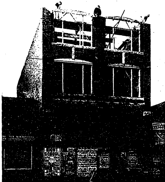
Business building for Bailley Bros., now being built on Eighth avenue east, Calgary, at a cost of $16,000. Dowler & Michie, Architects.
