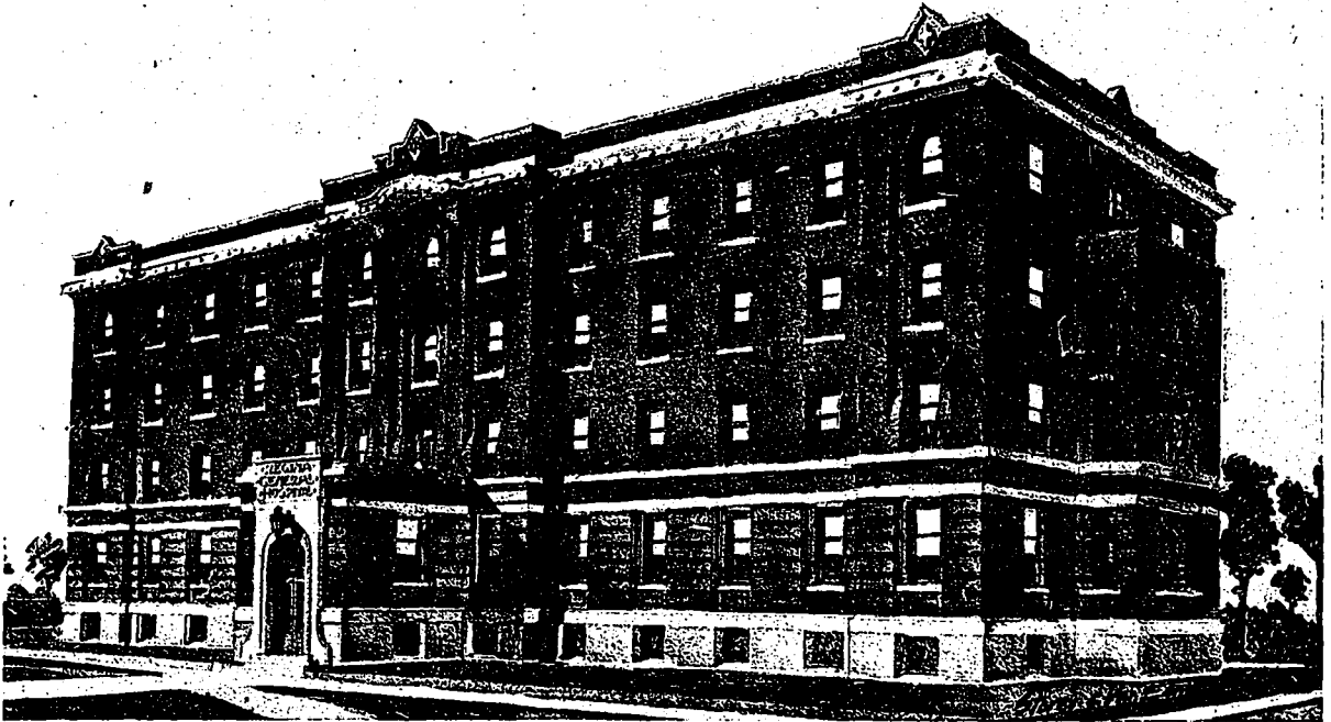
Regina's New General Hospital, now being built at a cost of $105,000. Although the building is to be entirely fireproof, in its construction, an additional precautionary measure is provided in an enclosed outside iron stairway, placed at end of the structure. Storey & Van Egmond, Architects.
