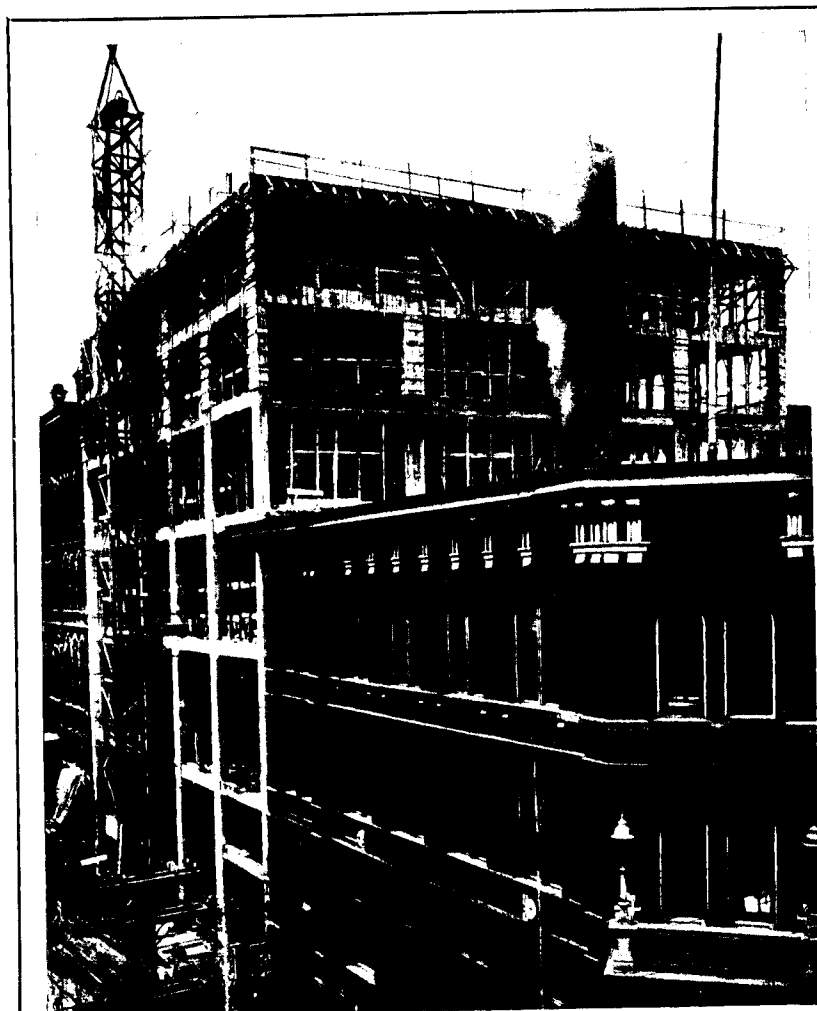
Cut shows Reinforced Concrete Building under construction for the Thomas C. Watkins Departmental Store, Hamilton.
