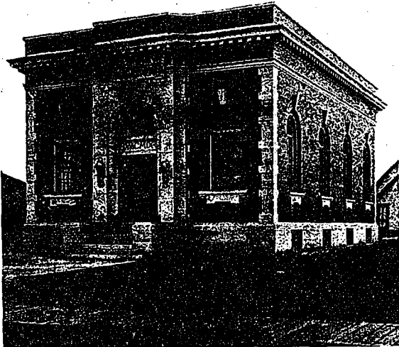
Land Titles Building, Saskatoon, said to be the most thoroughly built fireproof structure in Western Canada. It is constructed of dark brown clinker brick, with Tyndall stone trimming, the floor and roof being concrete, the partitions hollow tile, and the doors and windows of the most approved fire-resisting type. Storey & Van Egmond, Architects.
