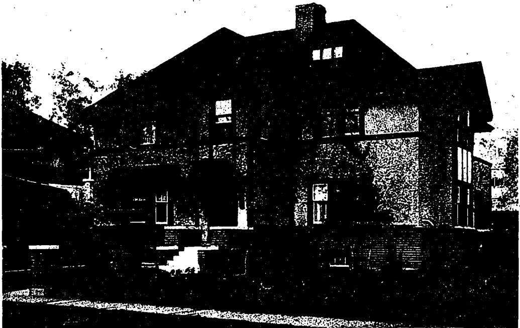
Residence of Mr. F. Christie, Betourney street. One of Winnipeg's many cement stucco houses, in which the plaster is applied directly to metal lath, thus making it a durable and permanent type of construction. J. D. Atchison, Architect.
