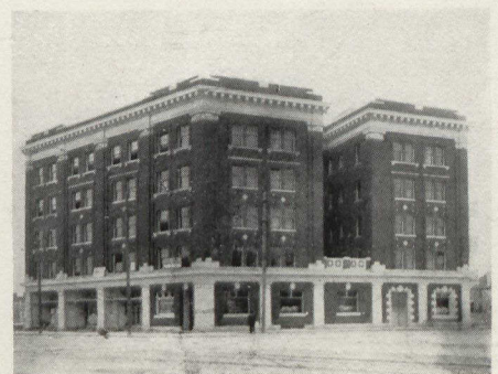
Casa-Loma Apartments, Winnipeg. J. H. G. Russell, Architect.
