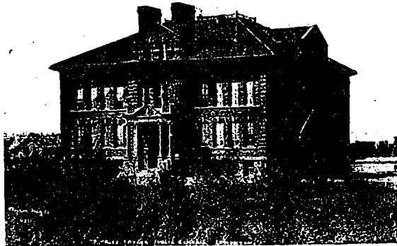
Alex. Taylor School, Edmonton. Roland W. Lines, Architect.
