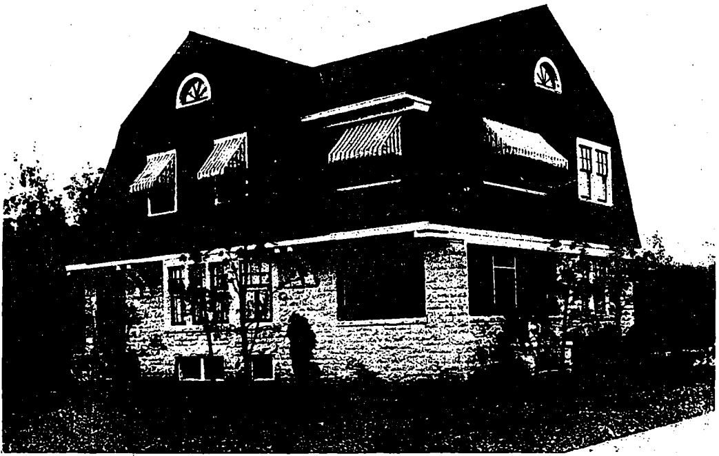
Home of Dr. K. C. Campbell, Ruskin Row, Winnipeg, an interesting example of a mansard-roof residence in which Tyndall stone and stained shingles are attractively combined. J. D. Atchison, Architect.
