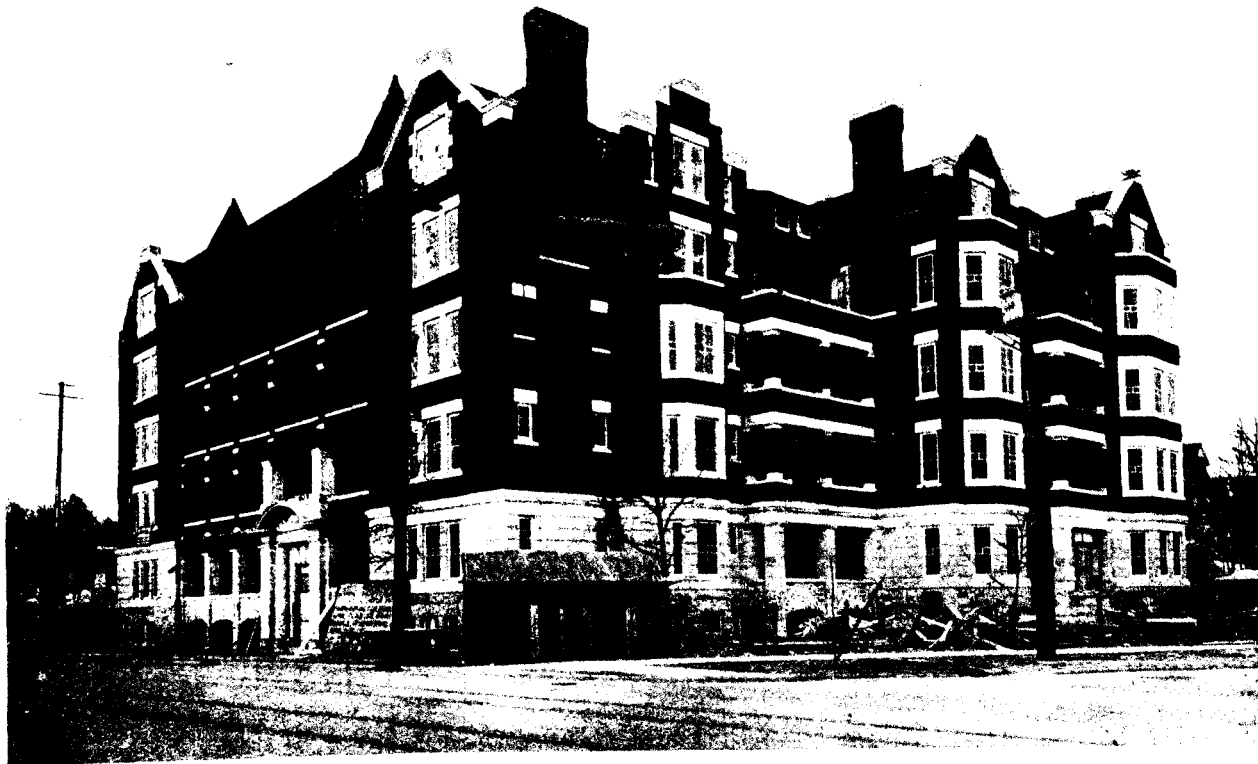
Roselyn Apartments, Winnipeg. R. J. Mattice, Owner. W. W. Blair, Architect. All the materials used in the construction of this building were supplied by us.
