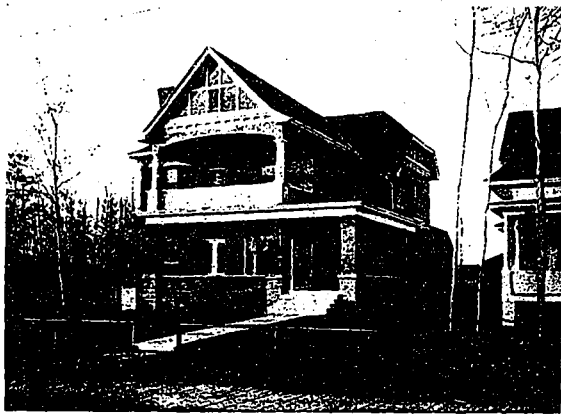
Residence of G. W. Swaisland, Victoria avenue, Edmonton. A. M. Calderon, Architect.
