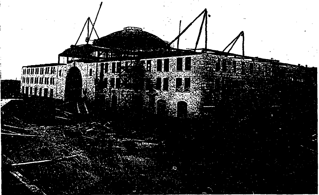
Fort Garry Station, showing the work well under way. When completed, Winnipeg will have the most modernly equipped terminal on the American Continent, if not in the entire world. Warren & Wetmore, Architects and Engineers.
