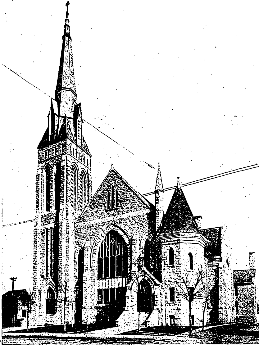
Augustine Presbyterian Church, built of Tyndall blue stone. One of Winnipeg's new ecclesiastical edifices. J. H. G. Russell, Architect.
