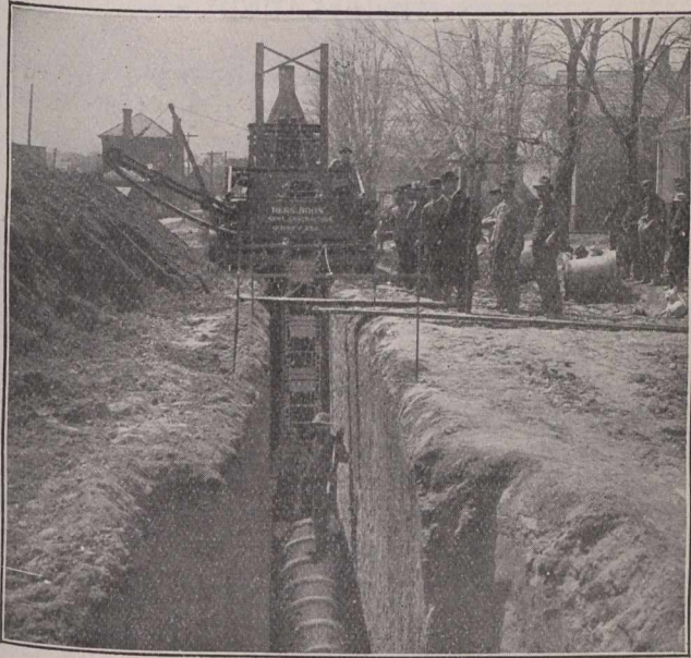
PARSONS EXCAVATOR - QUINCY, ILL.
