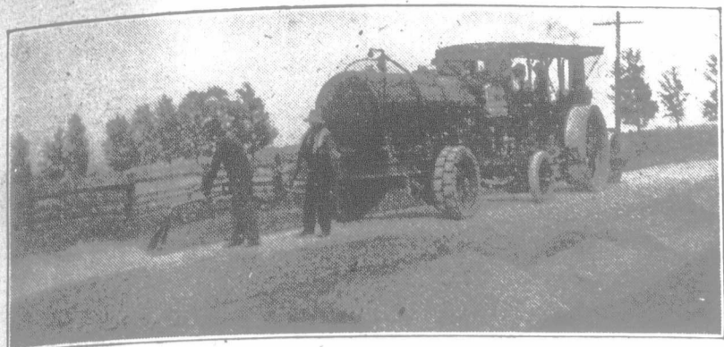
Applying "Tarvia-X" on Kennedy Road, Scarboro Township, Ont. Toronto & York Roads Commission.
