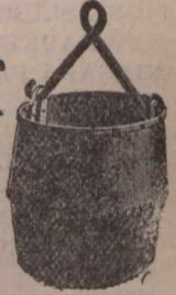
62—Mining Ribble with or without Valve in bottom
