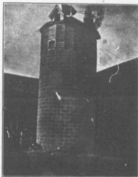
Cement Silo on A. C. Hallman's Farm
