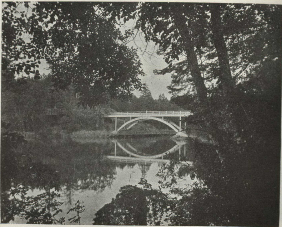
Gorge Bridge and Park, Victoria, British Columbia
