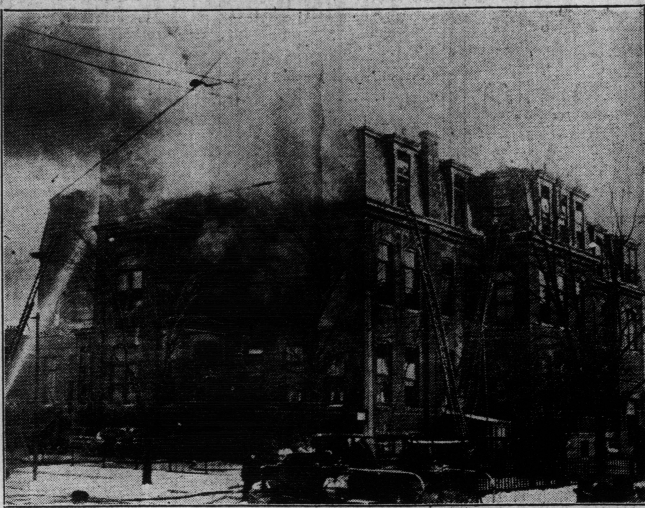
One of the oldest schools in the city, erected in 1886, and containing 20 rooms, was totally destroyed by fire yesterday afternoon. It was situated on the west side of Spadina crescent. The fire started at 3.40, shortly after most of the children had left the building. The remainder marched out in line without a sign of panic.
