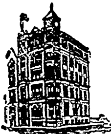
HEAD OFFICE BUILDING, MONTREAL.
