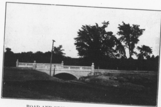
ROAD AND BRIDGE IN FRONT OF STATION.
