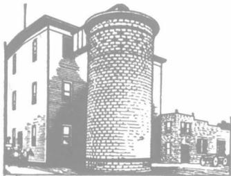
Grain Bin, built of Ideal Concrete Blocks, for The Marine City Roller Mills Co. Capacity, 5,500 bushels of wheat. Cost complete only \$860.
