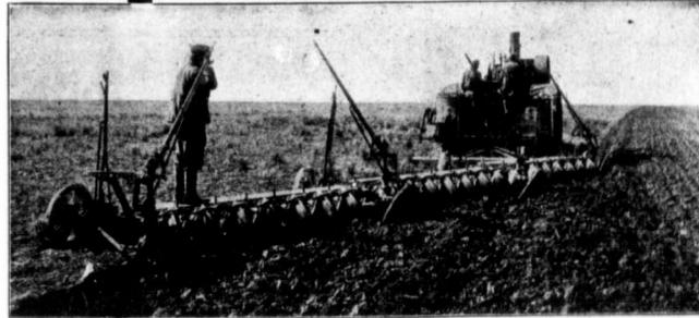
This is the plow for double service, as either disc or moldboard bottoms may be used on the same frame.
