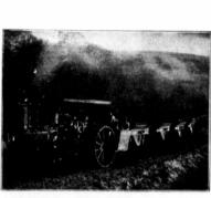
Big 4-30 gasoline tractor with self steering device, and an 8-bottom John Deere engine gang, using the full eight in stubble plowing, and only seven in breaking.
