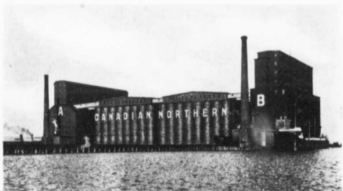
The Terminal Elevator of the Canadian Northern Railway at Port Arthur. Storage capacity 7,000,000 bushels; shipping capacity 250,000 bushels per hour.
