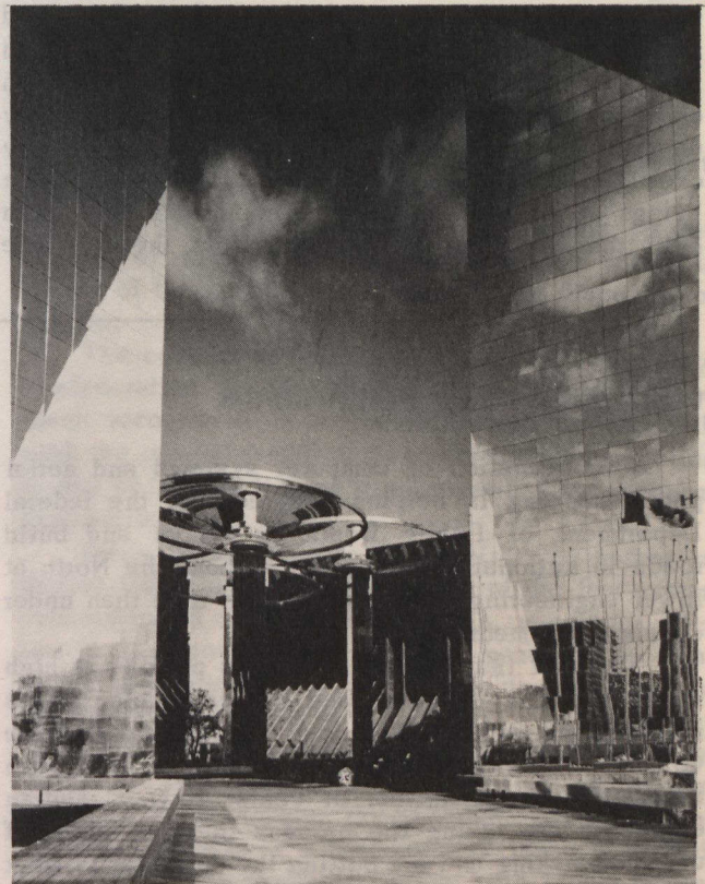
One of the entrances to the courtyard.
