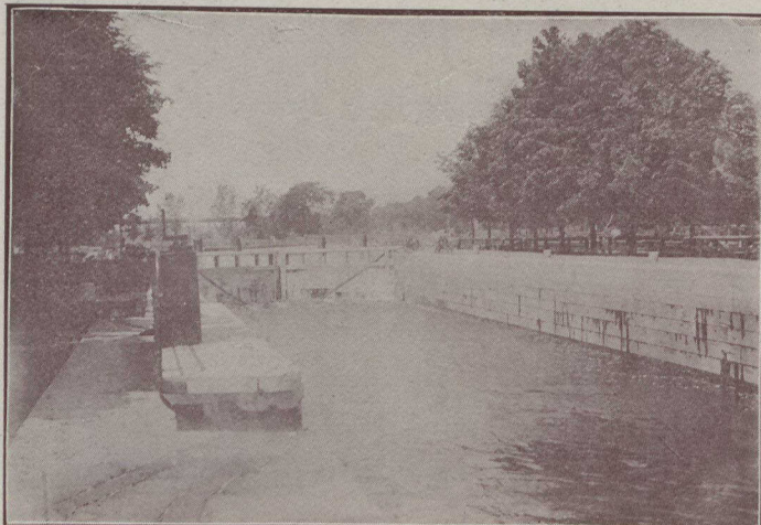
Canadian Canals Lock No. 6 on the Grenville Canal
