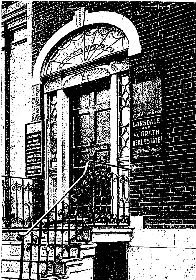
DOORWAY WITH SIDE AND FAN LIGHTS.
