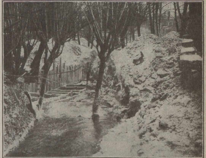
CREEK FLOW ENTERING BELLMOUTH—ICE ON BANKS IS EVIDENCE OF RECENT FLOOD
