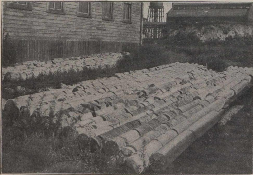
Part of 80 tons of Granite and Quartz taken from a 10-inch Bore Hole 2,000 feet deep by a Terry Class C. Drill. Some of the Cores are in solid pieces 18 feet long.
