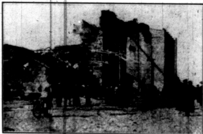
View of the Calgary Milling Company's Elevator during progress of Recent Fire.
