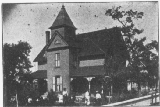
Postmaster Kerr's Residence, Oak Street.
