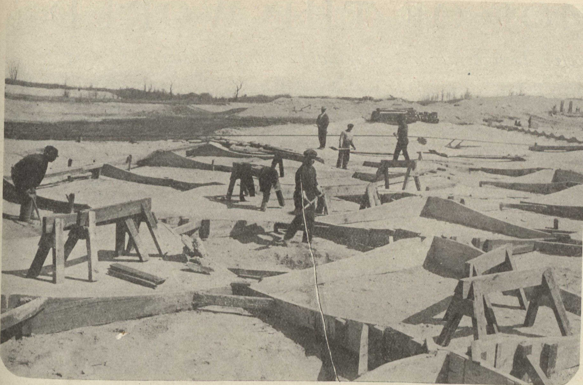
There are more than seven acres of Filtration Beds in the New Purification Plant now being built for less than a million dollars at Centre Island, Toronto.
