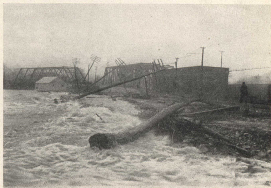
Telephone Poles undermined along the Shore of Humber Bay.
