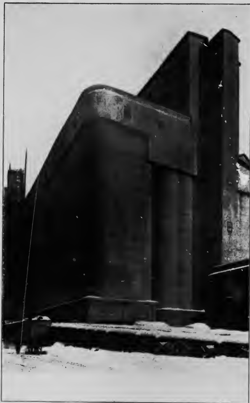
Harbour Commissioners' Elevator, Montreal.
