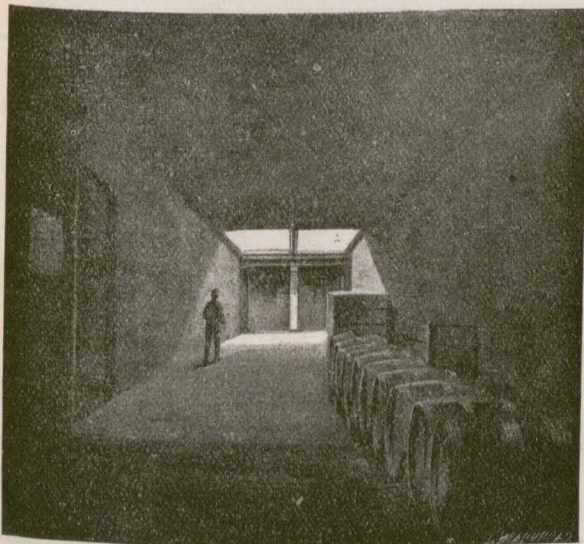
BASEMENT FITTED WITH ORDINARY SIDEWALK LIGHTS.
