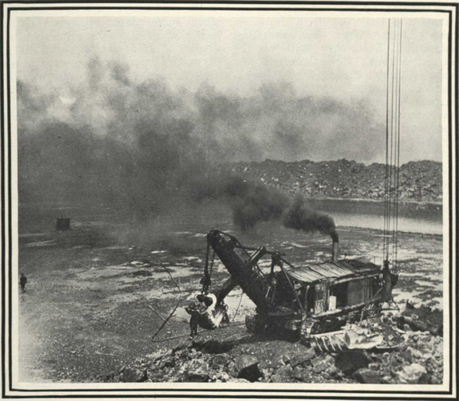
ANOTHER VIEW OF THE STEAM SHOVEL
