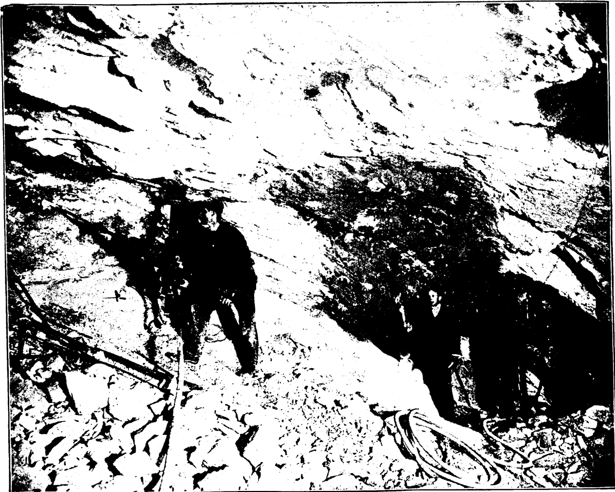
Two 2 \frac{1}{4} -inch Sullivan Drills working on 900-foot level of the Congress Mine, Congress, Arizona.
