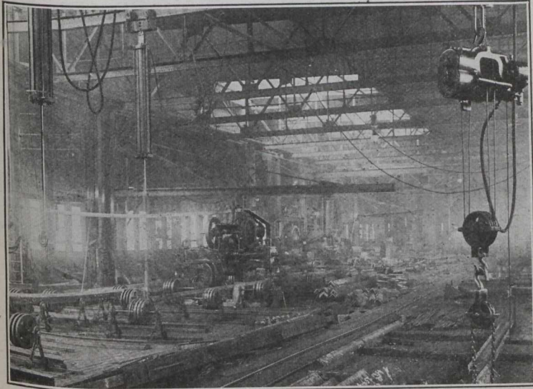
Interior view of Structural Shop No. 2. Taken from West Side.
