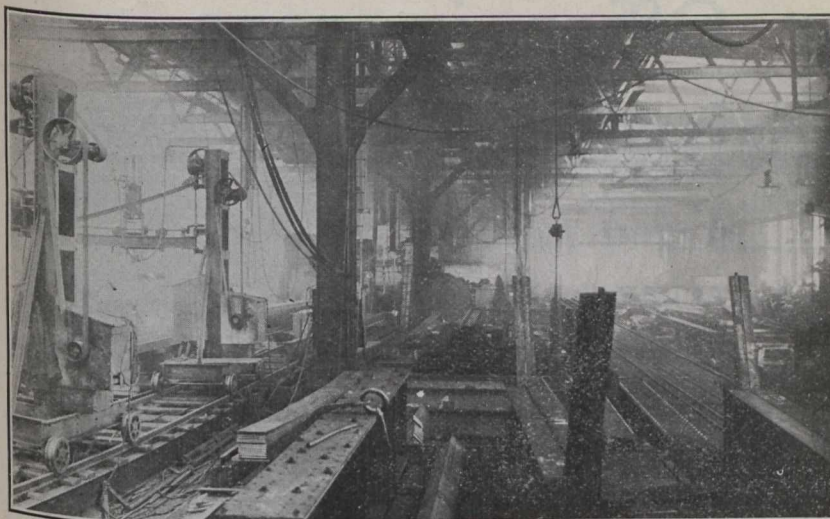
Interior of Structural Shop No. 2, Dominion Bridge Works. Taken from South East Corner.
