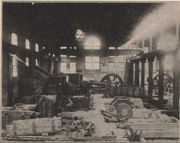
Shop Showing Traveller's Crane.
