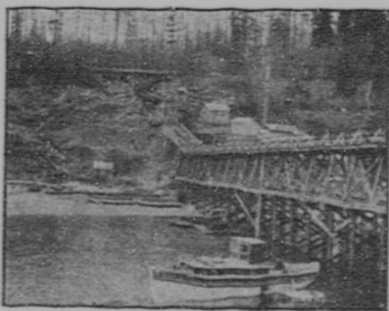
The wharf approaches also superstructure coal bunkers built for the Granby Co. at Russel Point, Ladysmith, by the Harrison, Lamond Construction Co., Ltd., 744 Hastings St., W., Vancouver, B. C. The supervising engineers consider this to be the best piece of construction of its kind in B. C.
