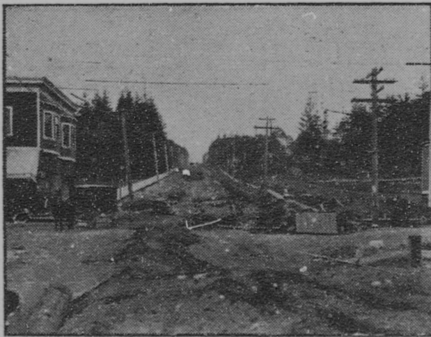
Grading Fraser Street before laying track, 1911
