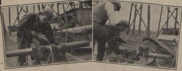
Cutting Crank-Shaft Welding Crank-Shaft
