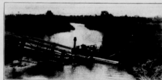
The wreck at Valley River Bridge, Boughen Bros. Outfit
