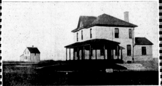
Superintendent's Residence, Nursery Station at Indian Head, 1915
