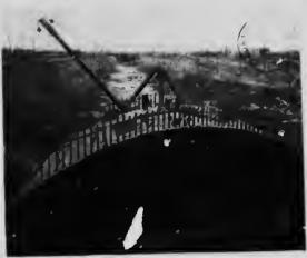
Centering for one of the concrete bridgee over the Chippawa power canal
