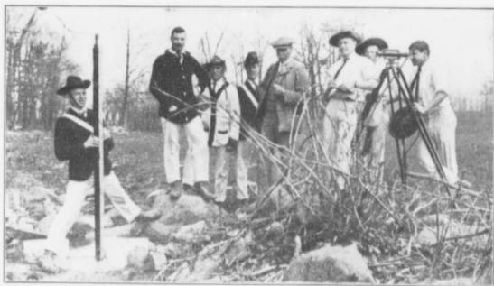
Civil Engineering.—Calculating the flow of a stream through a weir.
