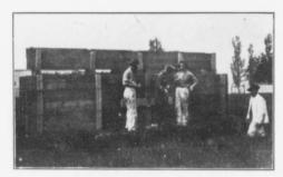
Laying the demolishing charge, of dry guncotton, on the side of the  $z^\prime$   $6^{\prime\prime}$  stockads.
