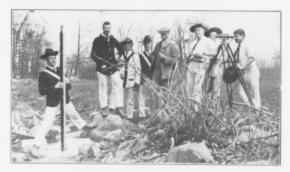
Civil Engineering.—Calculating the flow of a stream through a weir.
