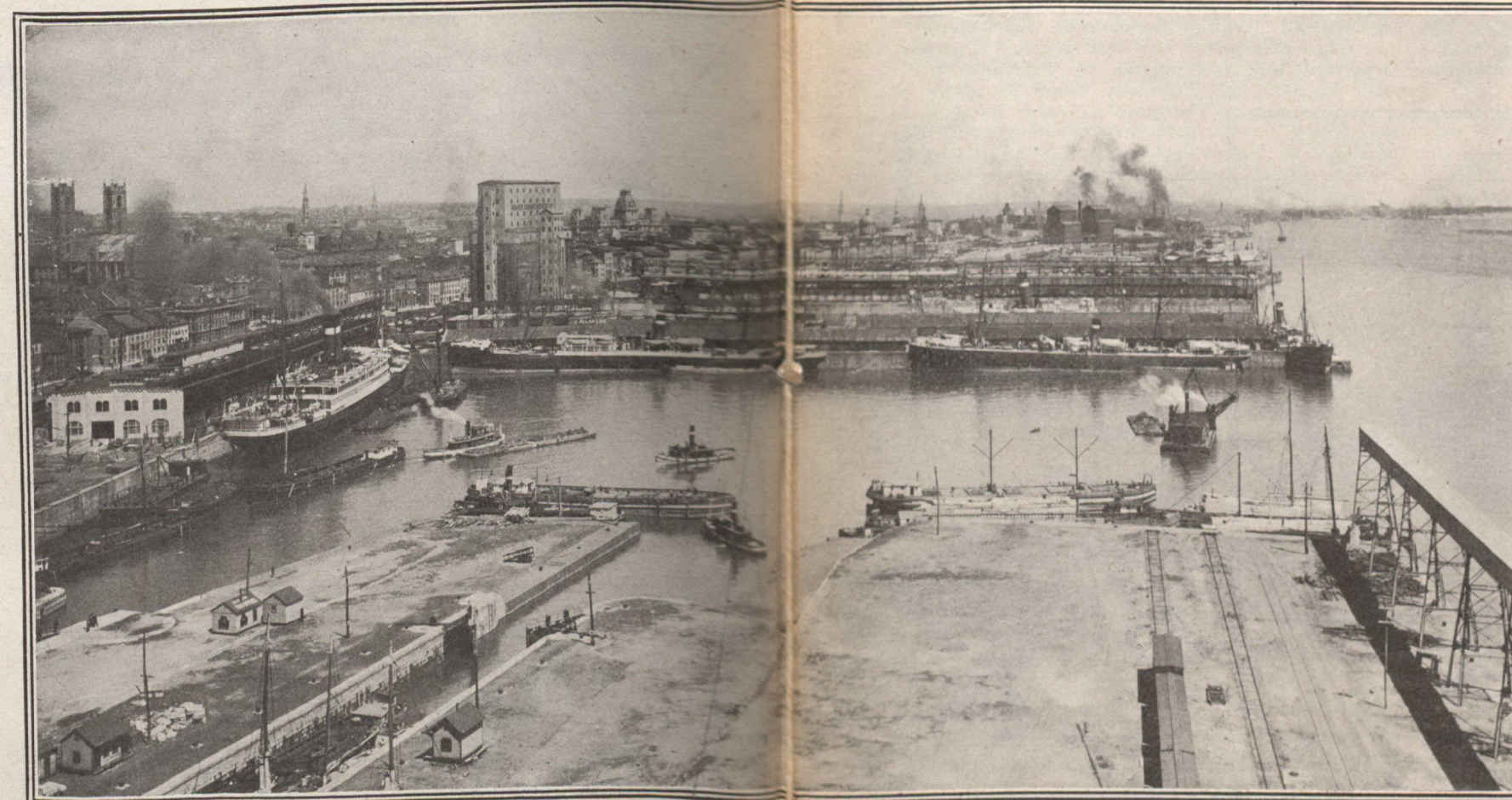
The furthest inland ocean port in America, Montreal Harbour is one of the finest harbours in the world. At present there is considerable rivalry between Montreal and Quebec City as to which shall get the new Government Dry Dock.
