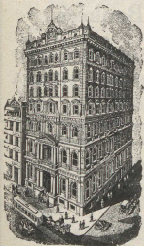
Head Office Building, Montreal
