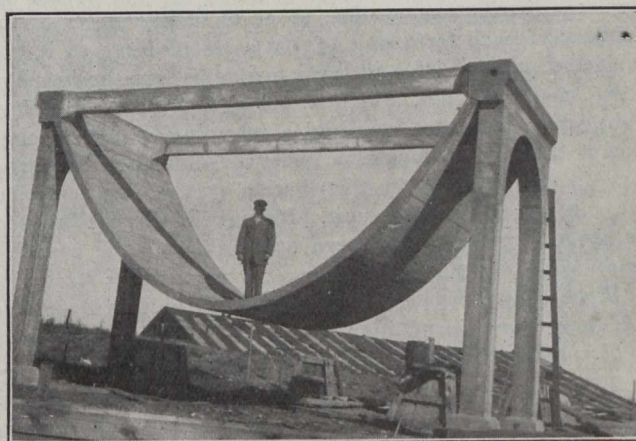
Fig. 11. Test Section, Proposed Aqueduct, 18 Ft. Wide, 9 Ft. Deep, 1,000 Ft. Long. Eastern Section of Irrigation Block.
