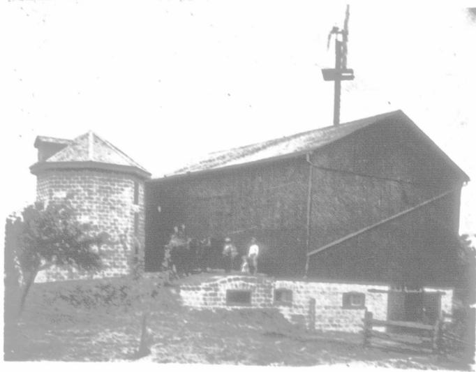
Size of barn basement walls 1 foot thick, 32 x 30 x 8 1/2, on an 18 x 18 inch footing. Used 65 bbls. CEMENT, and labor—2 men for 16 1/2 days. Size of root house 26 x 11 x 5 1/2, inside measure. Walls 1 foot thick, arch 10 inches thick. Is giving complete satisfaction. Size of silo 16 feet 8 inches inside diameter by 27 feet high. 18-inch walls at bottom, 11-inch at top. It has been filled to the top with corn cobs and husks from the canning factory, and has kept in good shape.
