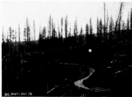
Flume on line of South Fork Canal.
