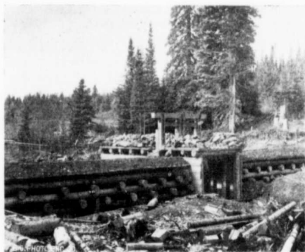
Dam at the Outlet of Bootjack Lake Reservoir.
