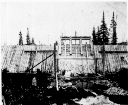
Discharge Gates in Dam of Morehead Pooling Reservoir.
