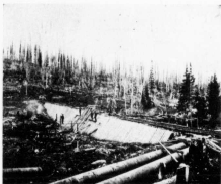
Rock Fill Cedar Crib Dam of Pooling Reservoir, at the delivery end of the Morehead Canal.
