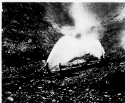
Two 8-inch Streams at work Washing Gravel from Lower Bench in advance of old Chinese workings.
