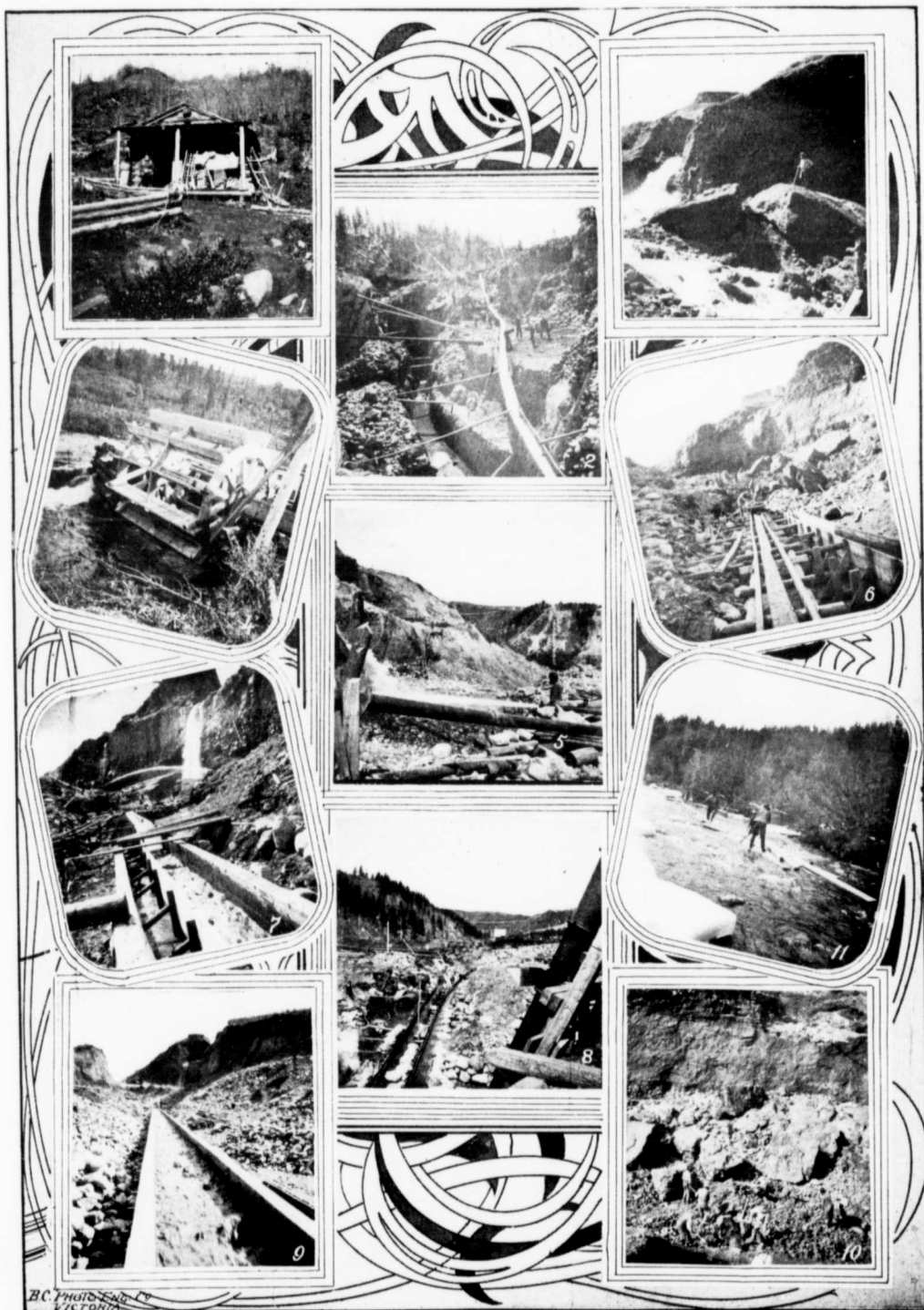
MINING IN Omineca. 1. Miner's Cabin on Lost creek. 2. Workings on Lost and Manson creeks. 3. Blasting boulder clay on Blackjack creek. 4. Undershot Wheel on Germanen creek. 5. Monitor at work on Manson creek. 6. Tramway for transporting foulders. 7. A pit on Blackjack. 8. Hydraulic elevator and workings, Kildare Gulch. 9. Arctic Slope Co's flume. 10. Blasting and picking clay. 11. Rafting lumber on Manson.
