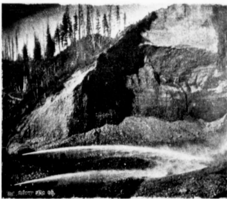
Two 8-inch Streams at work on the Upper Bench, washing Gravel from bank 350 feet high.
