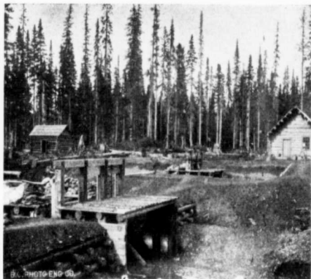
Dam Gates and Camp on Six-mile Creek, below Polleys Lake Cut.
