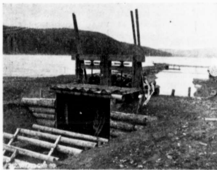
Jetties and Gate at the Outlet of Polleys Lake Reservoir.
