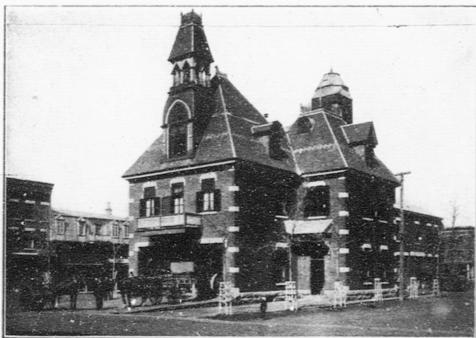
Station de Pompes.
