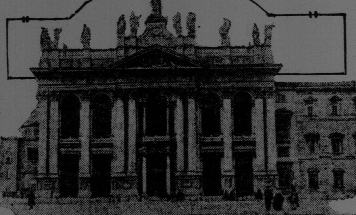
Church of St. John Lateran in Rome, one of the magnificent buildings which suffered damage in the earthquake. Several of the statues were broken and the building, which had undergone extensive repairs recently, was cracked in places.
