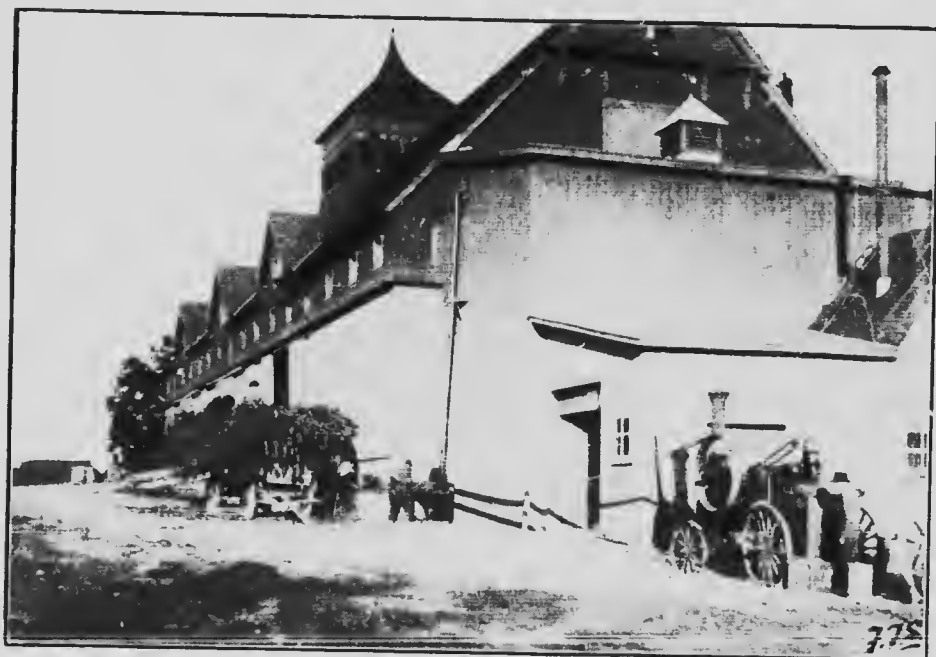
No. 10. Cutting into the Silo.
