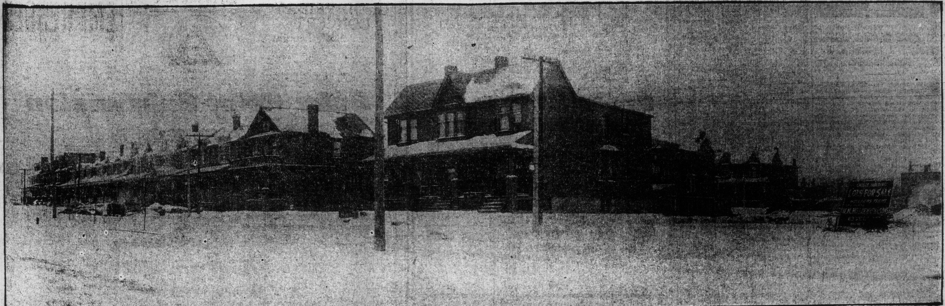
PHOTO TAKEN ON SAME SPOT ON JONES AVENUE, DECEMBER 21, 1912—SHOWING ELEVEN MONTHS' DEVELOPMENT WORK.
