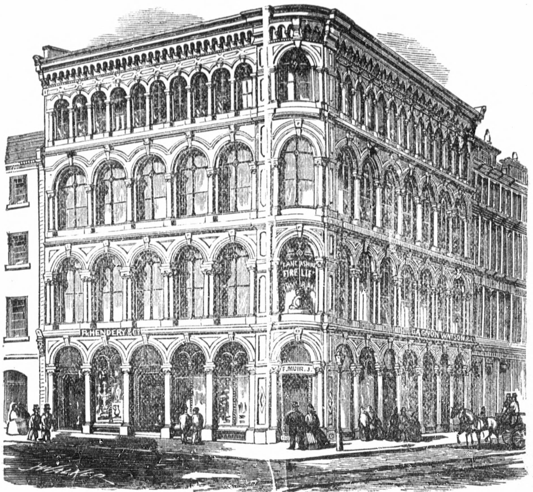
MUIR'S BUILDING, Notre Dame Street.
