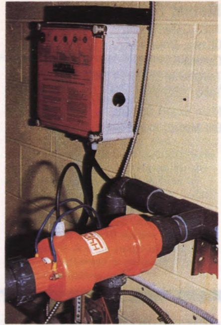
A commercial Hypocell System showing the control panel and monitoring support systems.
